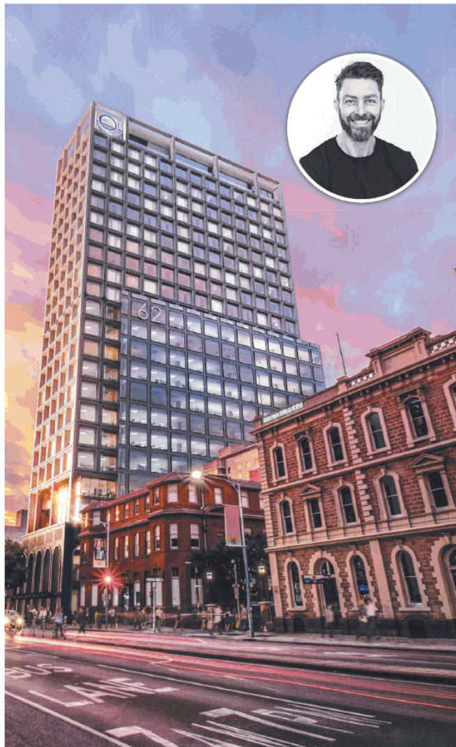
PARTNERSHIP: Work Club, which opened its first co-working space in Sydney in 2013, has agreed to take two floors in Axiom Properties' SIXTY2CURRIE project and, inset, Work Club founder and chief executive Soren Trampedach.
